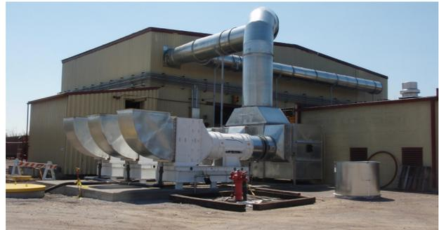
This Finn-designed system uses three Engart dust extractors operating in parallel to deliver 100,000ft<sup>3</sup>/minute of exhaust ventilation.
