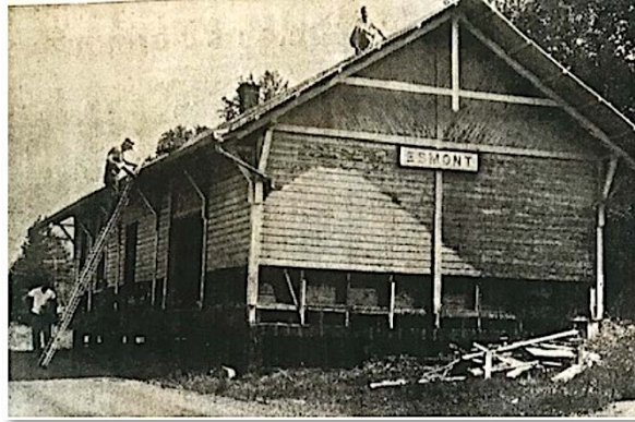
Esmont Depot Being Dismantled, 1964
