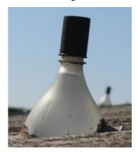
Take a 2l clear clean plastic bottle fill it 1/2 with water. Add 2 cupfuls' of bleach to stop Algae from growing. Top up bottle with water to rim & put on cap. The lamps work best with a black cap. Make a hole in roof. Push bottle through hole, cap 1st. Seal hole with polyester resin. Enjoy light without any energy bills. No electric shocks.
