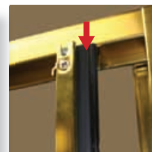
Bubble Seal Between Panel
