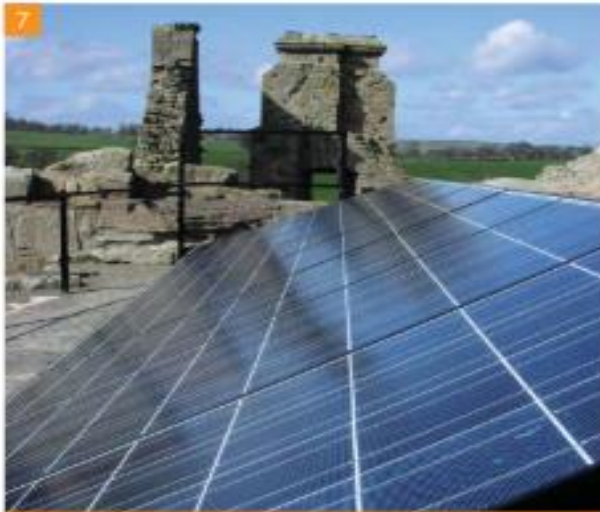
PV installation on a flat roof at Crichton Castle, which is now in the care of Historic Scotland (Photograph courtesy of Historic Scotland)
