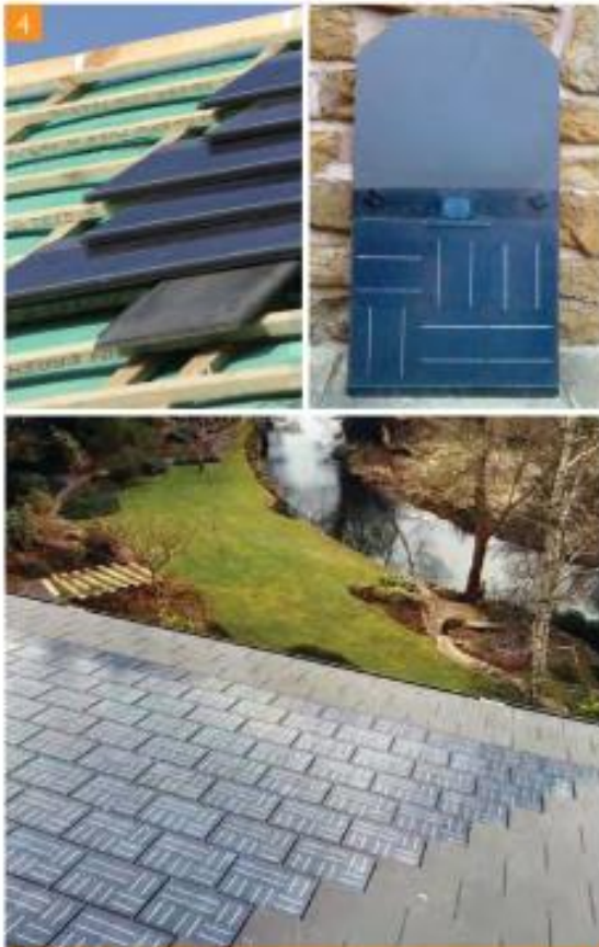
Top left: Close up of PV slate installation. Top right: Individual PV slate. Bottom: Roof covered with PV slates. (Top left and bottom: Photographs courtesy of Saralata Limited. Top right: Photograph courtesy of Solar Century.)
