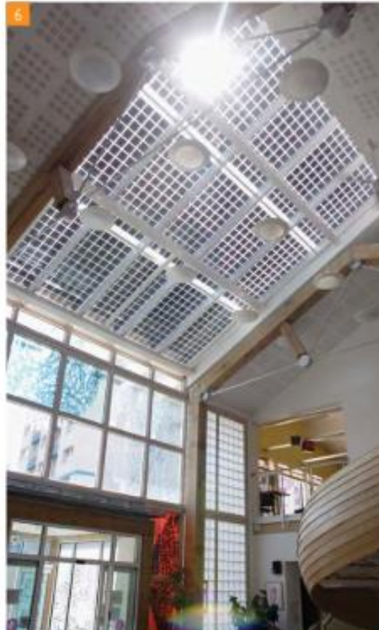
PVs integrated into glass (Photograph courtesy of Solar Century)
