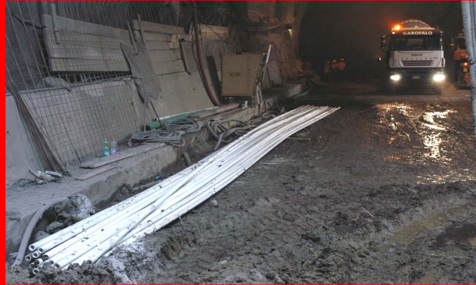
PHASE 2: Positioning pipes
