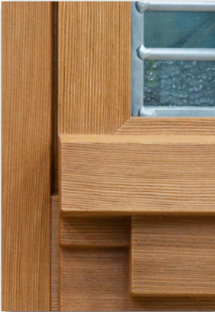
Details of the Craftsman Fir Grain Construction
