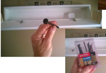
We reccomend flat head torque screws as show. Use a stud finder to find location of wood wall studs. Then attach unit to wall stud with screw. Use a level to adjust before adding additional screws to minimum of three studs.
