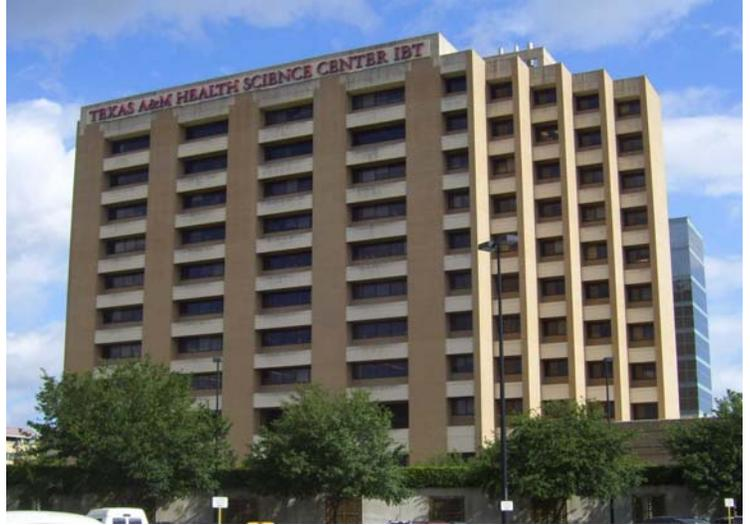
The IBT is an eleven-story concrete frame office building and an adjacent two-story laboratory wing constructed around 1989. The exterior walls are constructed with brick masonry veneer and CMU backup walls, precast concrete spandrel beams and sunscreens, and aluminum framed windows.
