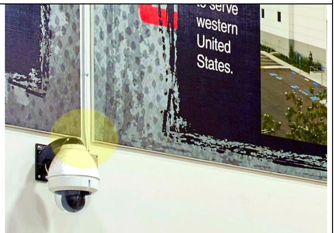
TS32 Frames-Gym Court-Zoom on Corner & Graphic fixed on the side
