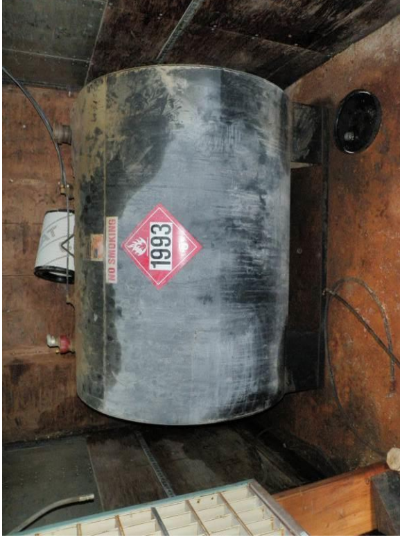
2. One 300-gal (approximate) diesel/fuel oil AST – The fill gauge read approximately \frac{1}{4} full. Staining observed.
