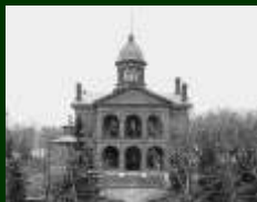
Front view, the Washington County Courthouse, Stillwater. Photographer: John Runk (1878-1964) Photograph Collection 5/16/1914 Location no. Runk 995 Negative no. Runk995
