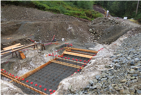
Powerhouse footing rebar
