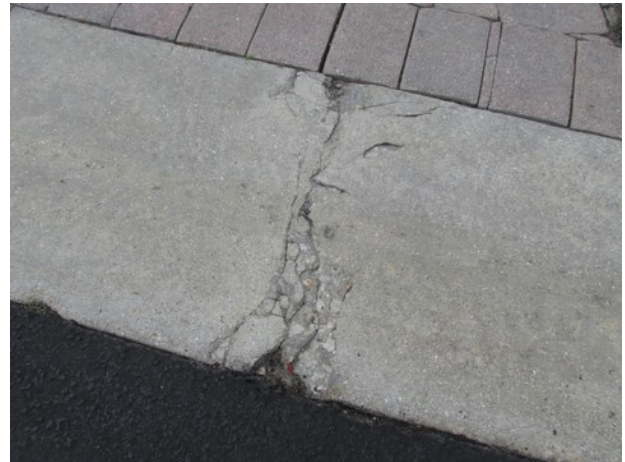
Gutter crack at 3308 Turtle cove
