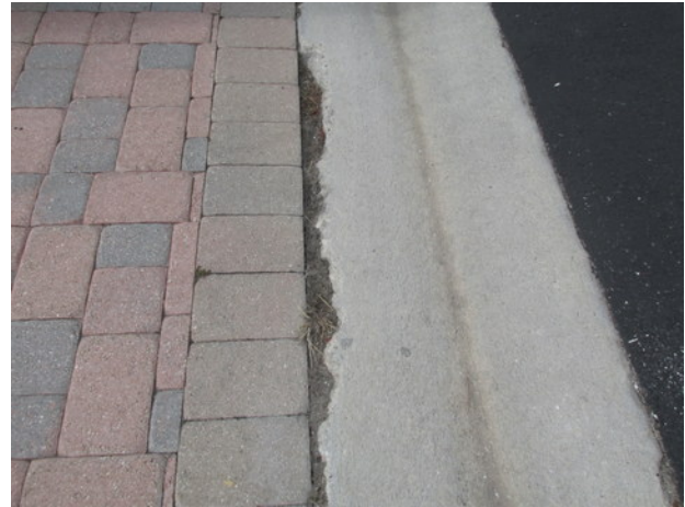
Gutter edge deterioration at 3163 Turtle Cove
