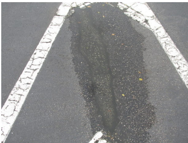
Pavement deterioration
