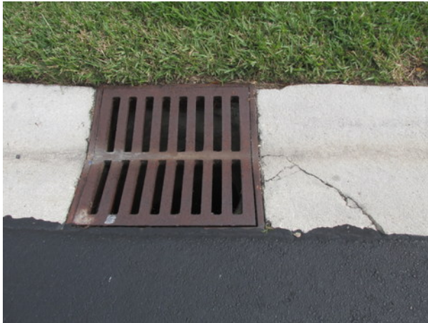
Typical catch basin with minor settlement
