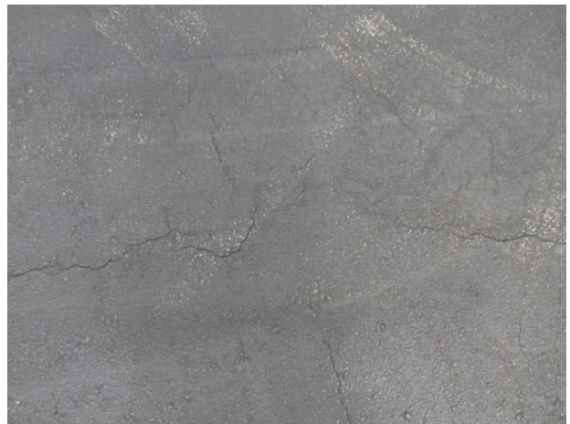
Pavement cracks
