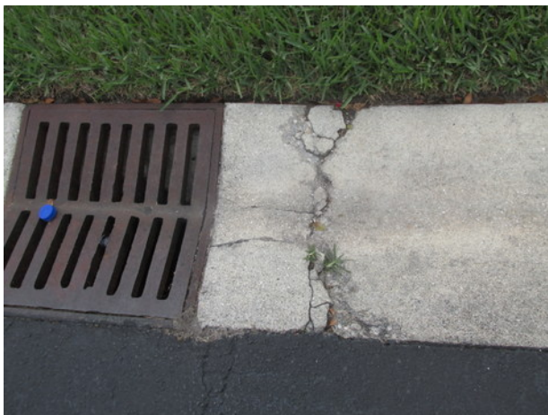
Gutter crack at 3344 Turtle Cove
