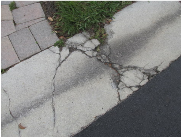
Gutter Cracks at 3382 Turtle Cove
