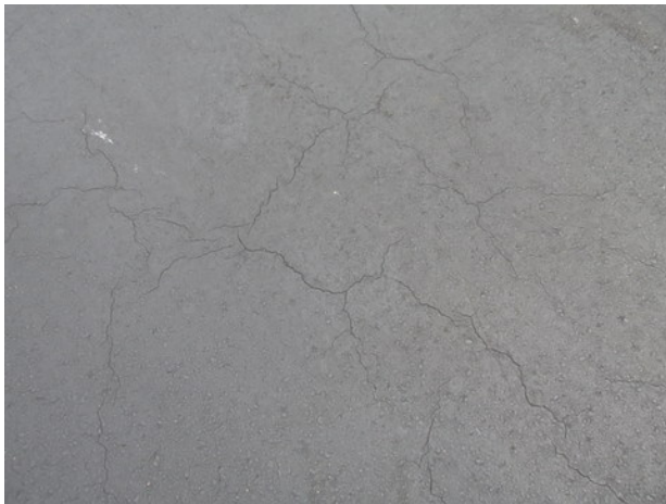
Pavement cracks
