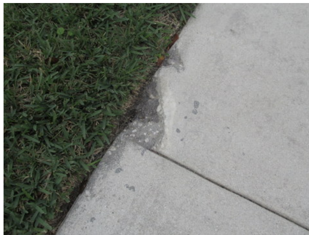
Sidewalk edge deterioration at 3302 Turtle Cove
