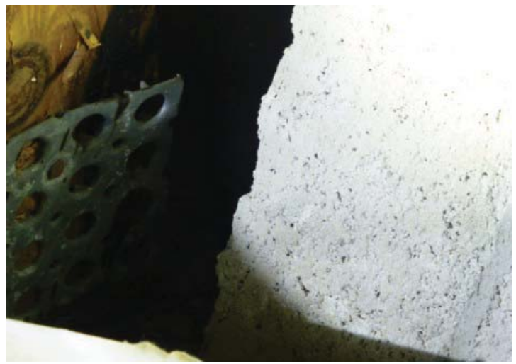
#4 ROOF TO WALL ATTACHMENT OPPOSITE SIDE
