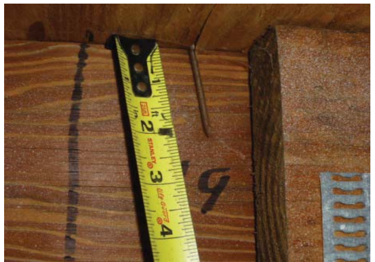
#3 ROOF DECK ATTACHMENT
