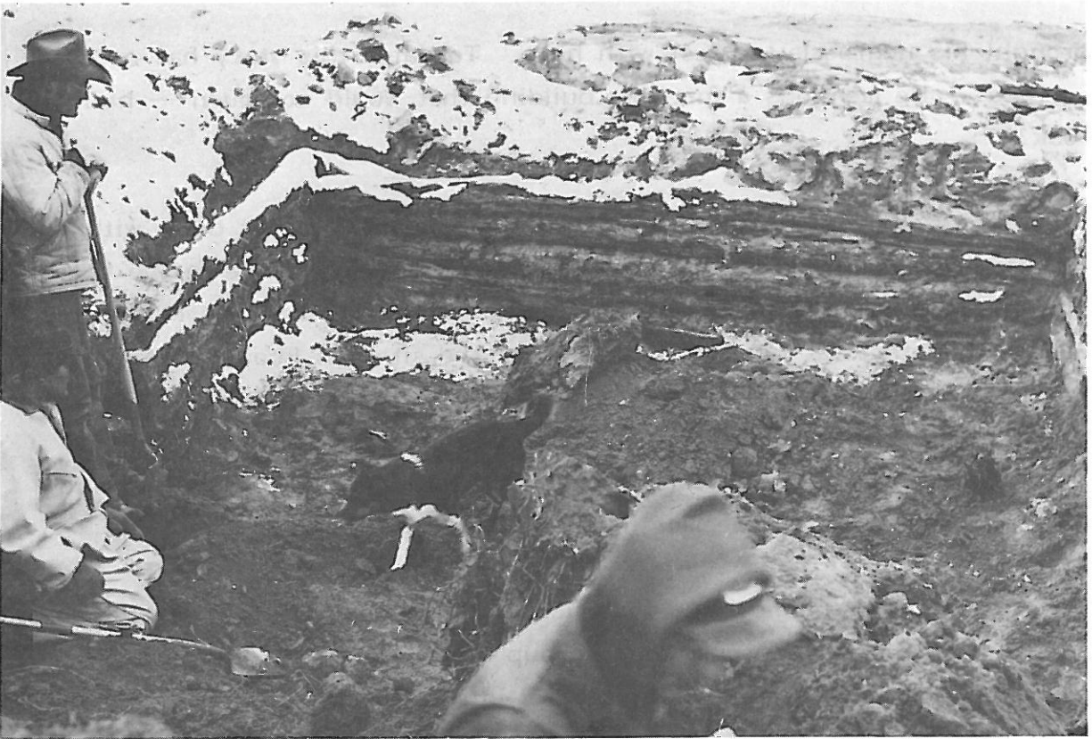
Foundation and log sub-wall of No. 1 Rock Ranch.
