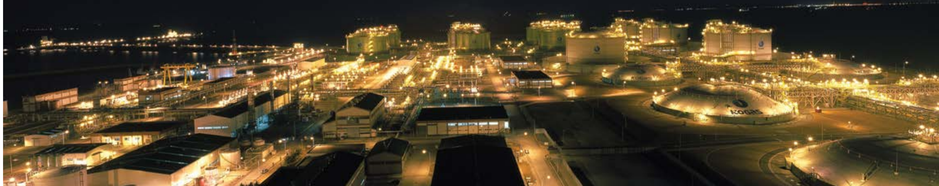
Incheon Terminal - Courtesy of KOGAS
