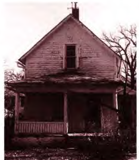
Simmons house on 27th Street
