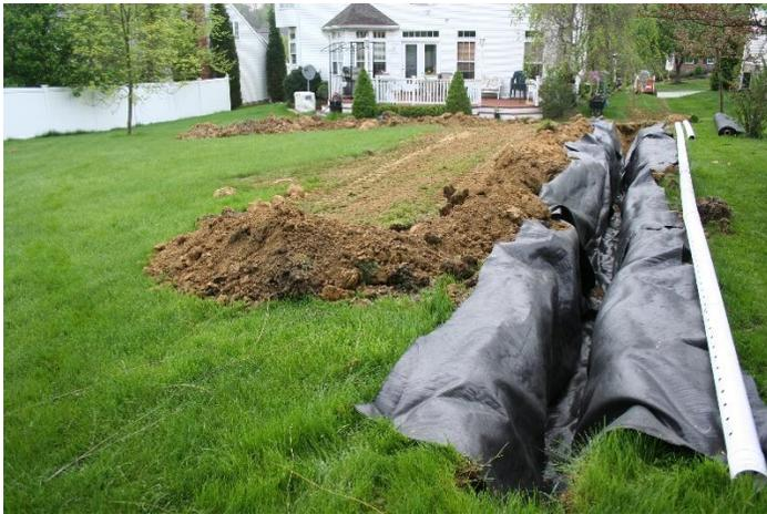
Perforated pipe covered with stone and wrapped in fabric
