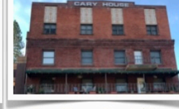
#9 Cary House Hotel: (The Hotel Placerville Building. Later called The Raffles Hotel) 300 Main Street. Built 1915 on the site of the original Cary House. In 1983 the building was remanded the Cary House Hotel.
