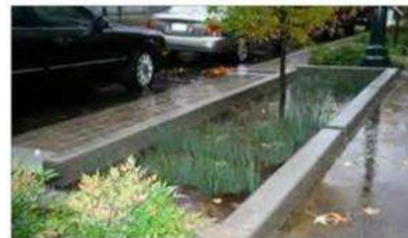
Curb cuts lead runoff water into landscaped rain gardens
