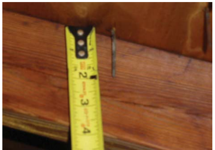
#3 ROOF DECK ATTACHMENT 8d NAILS
