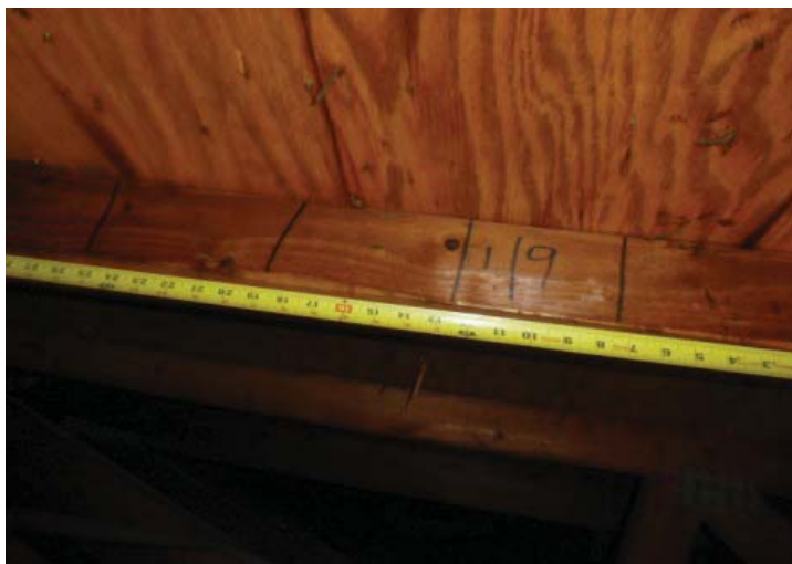
#3 ROOF DECK ATTACHMENT 6" X 6" NAIL SPACING
