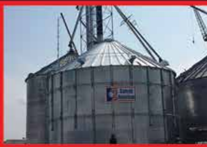
Grain Bin Construction and Remodeling
