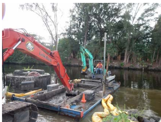
Excavator at boat ramp unloads barge
