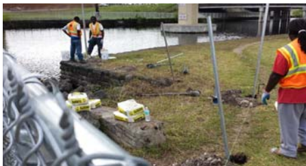
DOT Crew begins installation of fence in Nov.
