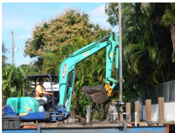
Bucket load of grainy sand material
