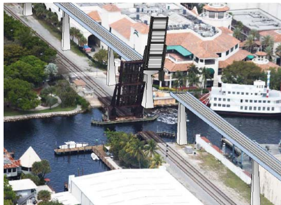
From the report: CONCEPTUAL RENDERING OF HIGH LEVEL MOVABLE PASSENGER RAIL BRIDGE AND VIADUCT OVER THE NEW RIVER.
