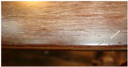
You boy's ready to get started sanding???????? I start with 100 and use it until I start to spray the first coat. Then its 600 wet dry. Final is 2000 grit wet dry. Here's a couple 1959 & 1960 all in different stages of work.
