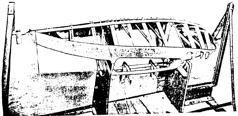
Figure 35 - Wing Tip Float Jigs
