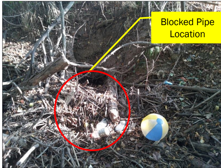
Debris and Sedimentation in/near Culverts
