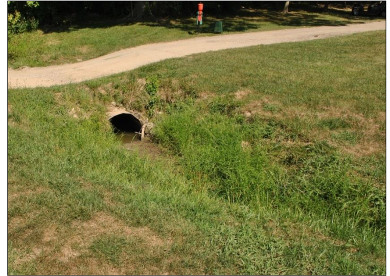
Debris and Sedimentation in/near Culverts
