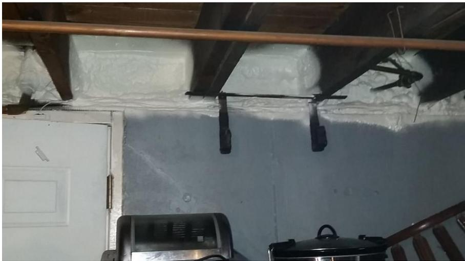
There are a couple different approaches to sealing up and insulating rim joists. The first approach is to use closed cell spray foam. Ideally we would install 2 to 3 inches of closed cell spray foam. This seals up the rim joists and stops air leakage. The other approach is to cut 2" polyiso foam board and fit it in between each rim joist. We then dense pack cellulose behind the foam board and seal around it with a hand held foam canister. This also stop the flow of air and insulates the area.
