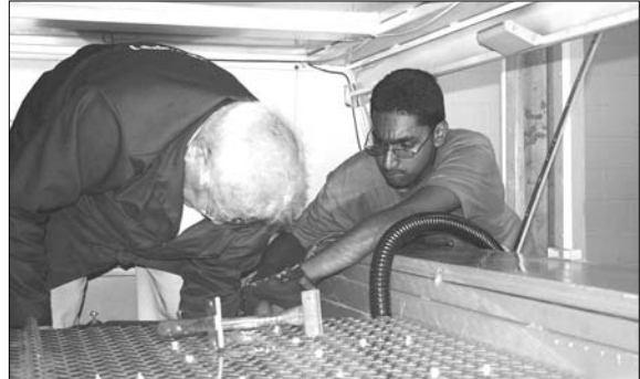
Paul Kydd and BCIT student helper Andrew Mohabir wrestle with the instillation of the GNB advanced sealed lead acid batteries.
