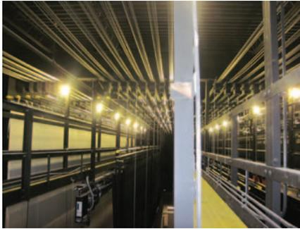
The stage catwalks at John Cooper School's PAC provide access for inspecting and servicing the rigging, which is not possible when it is simply underhung, yet does not restrict the travel and high trim below useful minimums, as a full stage gridiron would in a 50' high stage.
