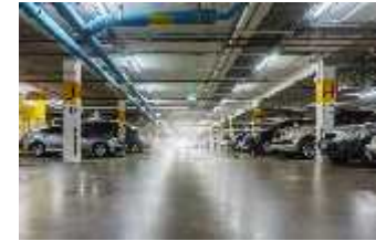
Enclosed Vehicular Facilities
