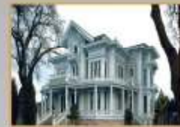
Standalone Access Control: House
