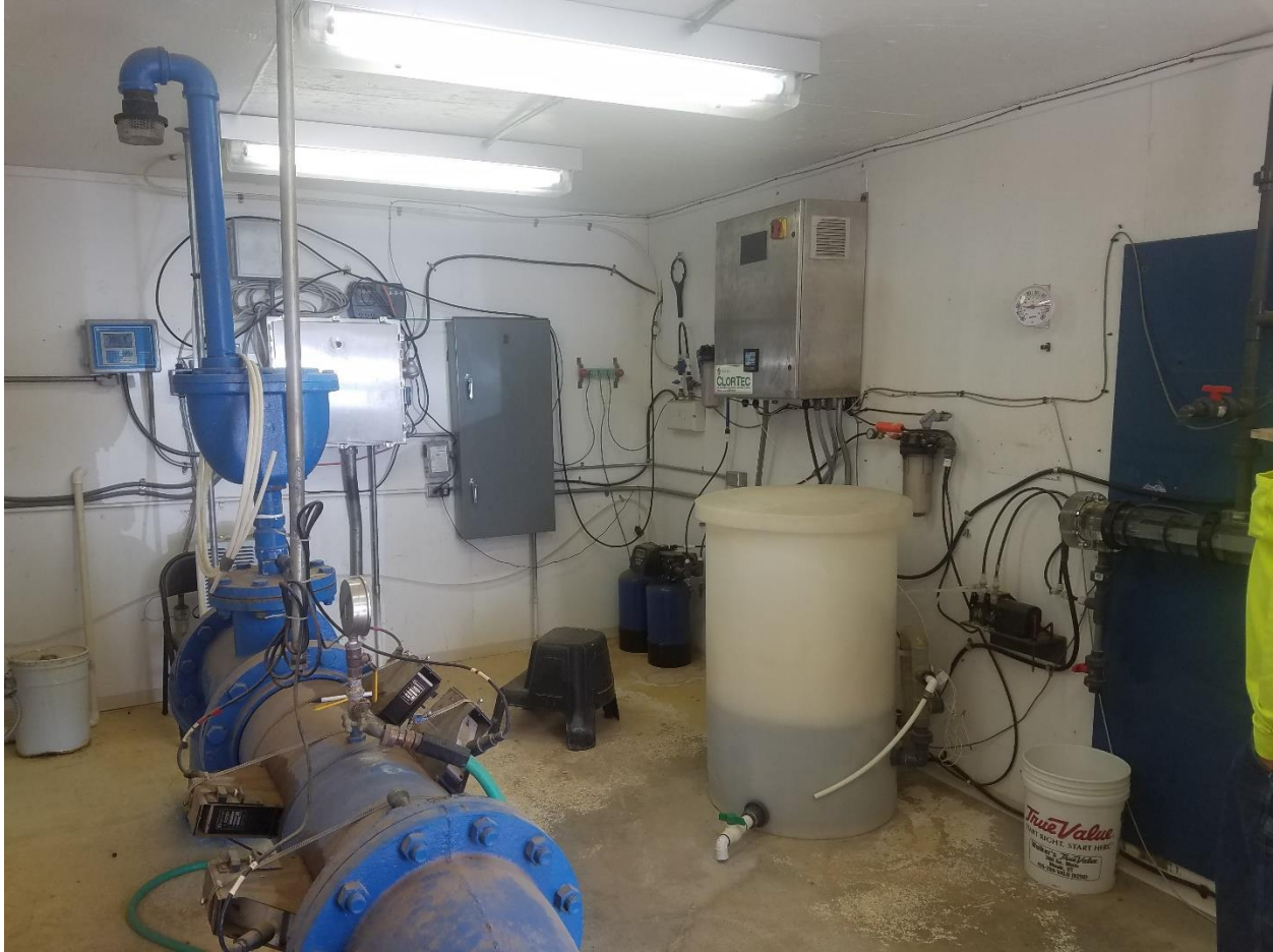
Figure 2 – Chapman/Spanish Valley Well Building
