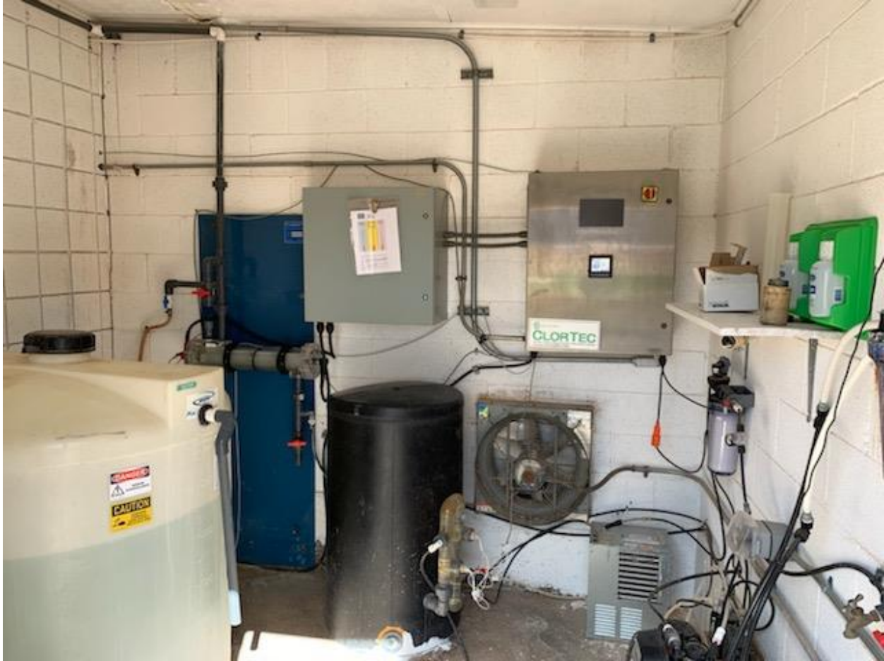
Figure 1 – George White Well Building
