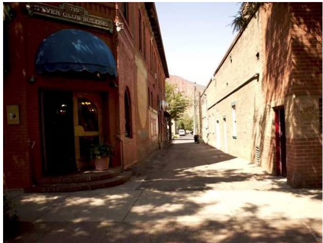
I- BEFORE: The alley running between Grand Avenue and Colorado Avenue in the 700 block, prior to the existing beautification efforts.
