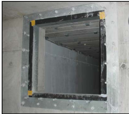
Figure 9 – Bolted Access Hatch
