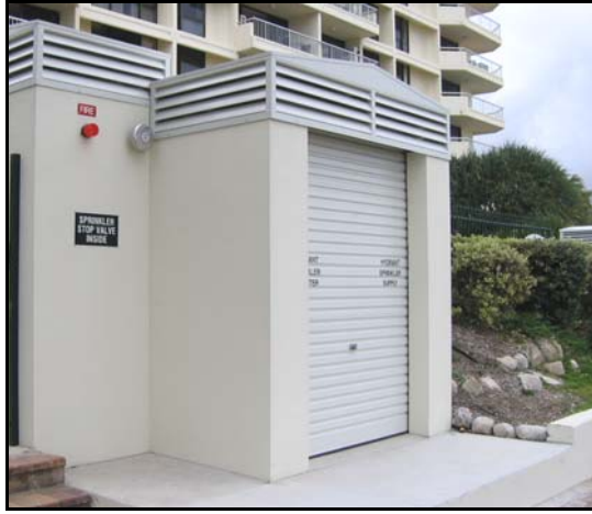
Figure 7 –Enclosure with Roller Shutter – referred to in Coolum Beach as “The Taj Mahal”
