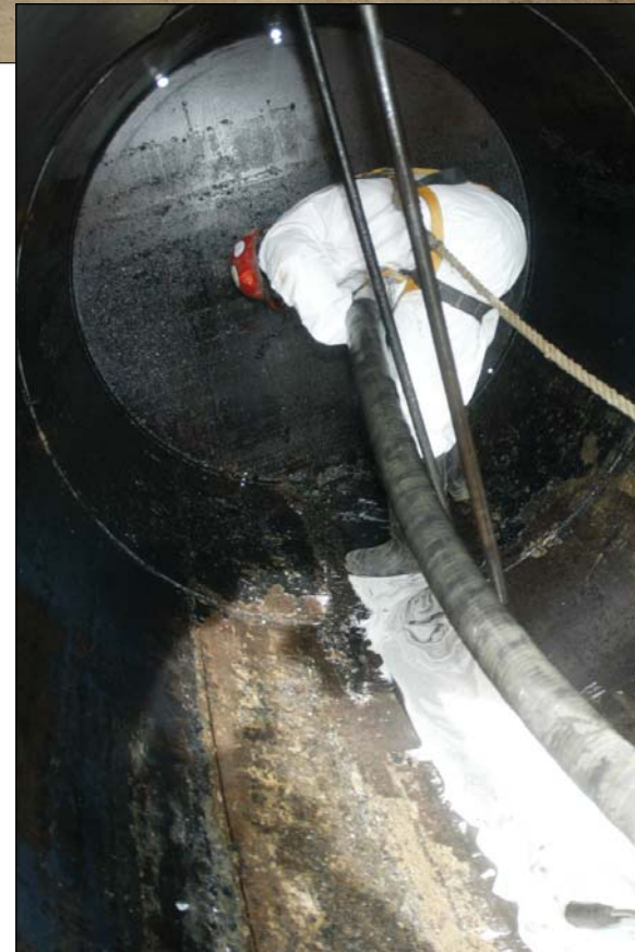
Top photo: Jeff Conger positions the 3,500-gallon International vacuum truck with aluminum tank at a site in Moline, Iowa. At right, Chris Kullas vacuums excess water and fuel from inside an underground storage tank that was dug up and pressure washed. Above, Conger assists Kulla as he exits the tank.
