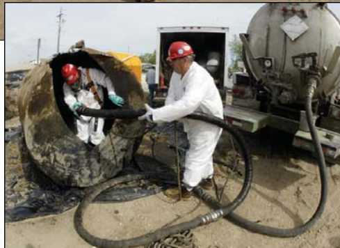
Top photo: Jeff Conger positions the 3,500-gallon International vacuum truck with aluminum tank at a site in Moline, Iowa. At right, Chris Kullas vacuums excess water and fuel from inside an underground storage tank that was dug up and pressure washed. Above, Conger assists Kulla as he exits the tank.
