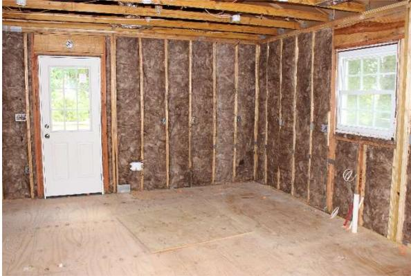
This is where the kitchen will be and, if you look closely, you can see the electrical wiring, the plumbing, the HVAC duct, the subfloor, the new kitchen door, the new kitchen window and the insulation are all done. The rest of Camp Centurion is in the same condition and the drywall is next.
