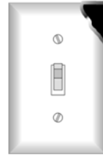
CRACKED OR BROKEN COVER PLATE
