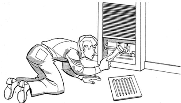
BURNERS AND HEAT EXCHANGER ARE CHECKED FOR DEFECTS
