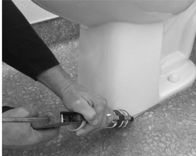
SEALER BEAD APPLIED AROUND ENTIRE BASE OF TOILET
