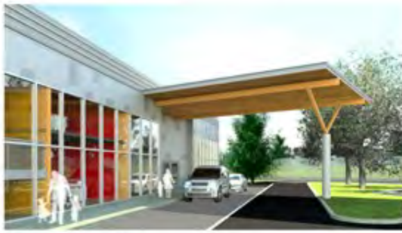
Figure 4.4.8.1 Entrance and Drop Off Area
