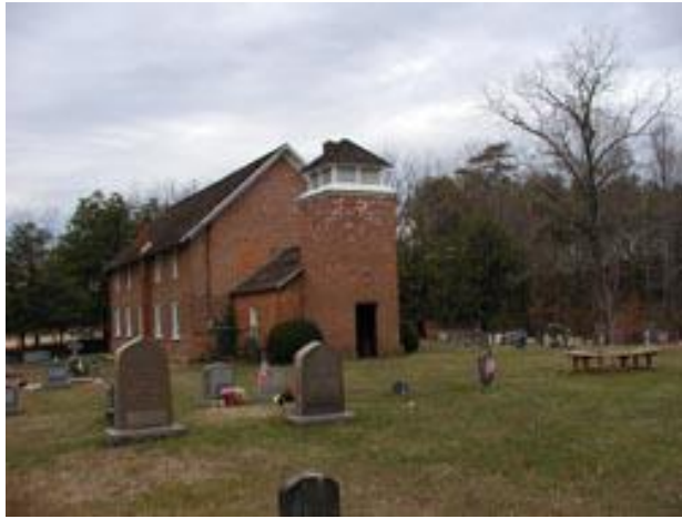
Rear of Church
