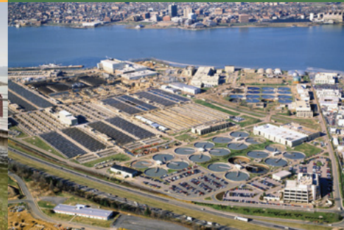
NEW DIGESTERS, BIOSOLIDS AND CAMBI PROCESS
