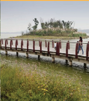
BOARDWALK AT ISLAIS CREEK
