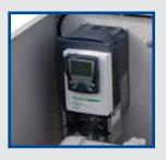
Variable Frequency Drive for constant pressure, variable flow and surge free soft starting
