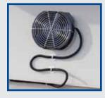
Exhaust fan cools the pump motor, switchgear and control logic. It activates when the pump starts.
