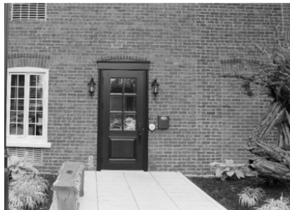
July 2017, now remodeled but door and wall still very visible
