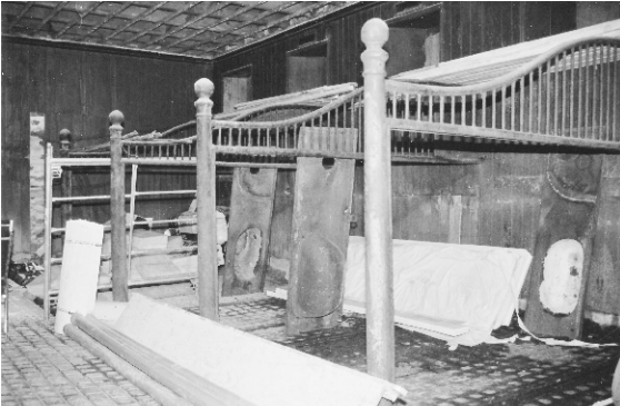
The stalls before the renovation in 1999
