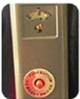
A manual reset control, the limit control's set point is at a higher temperature or pressure than the operating control.
