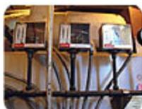
Pressuretrols determine the operating range of the boiler during the heating cycle.
