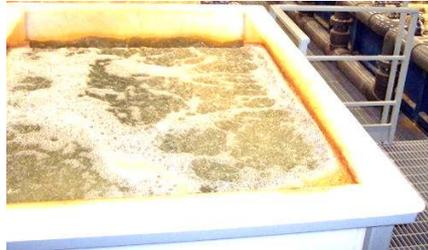
**Figure 4: 1,900 L/m Reaction Chamber**
