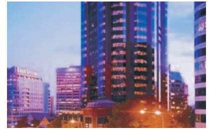
101, Miller Street, Australia 426 TR (1500 kW)
