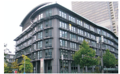
T Systems, Germany 41 TR (144 kW)
