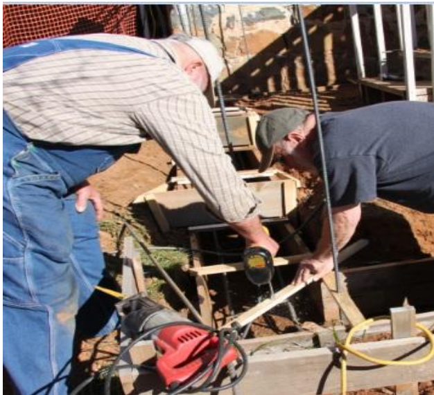
Rodney and Steve begin the new porch foundation
