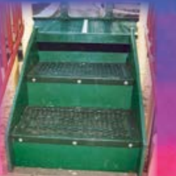
ADA Deck to Deck Steps
