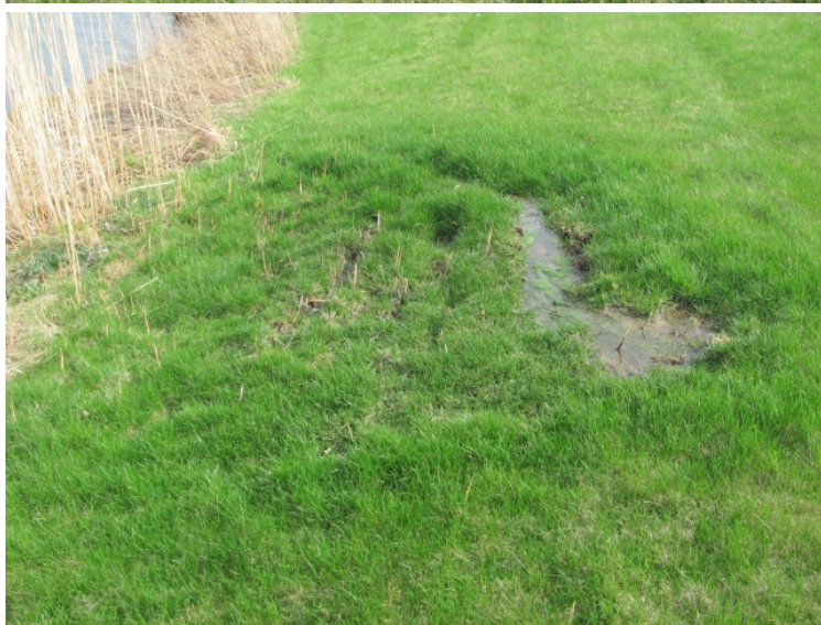
Erosion along west side of Stormwater Management Area South
