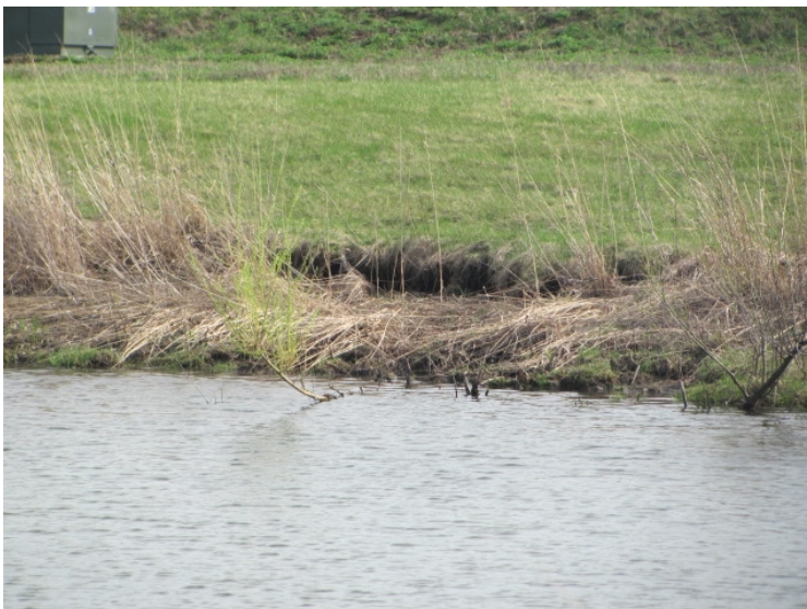
Shoreline erosion at south perimeter of Stormwater Management Area South
