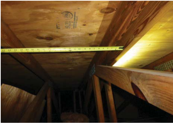
TRUSS/RAFTER SPACING
